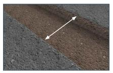
Confirm trench widths suitable: LONG SIDE 700mm. SHORT SIDE 400mm.
