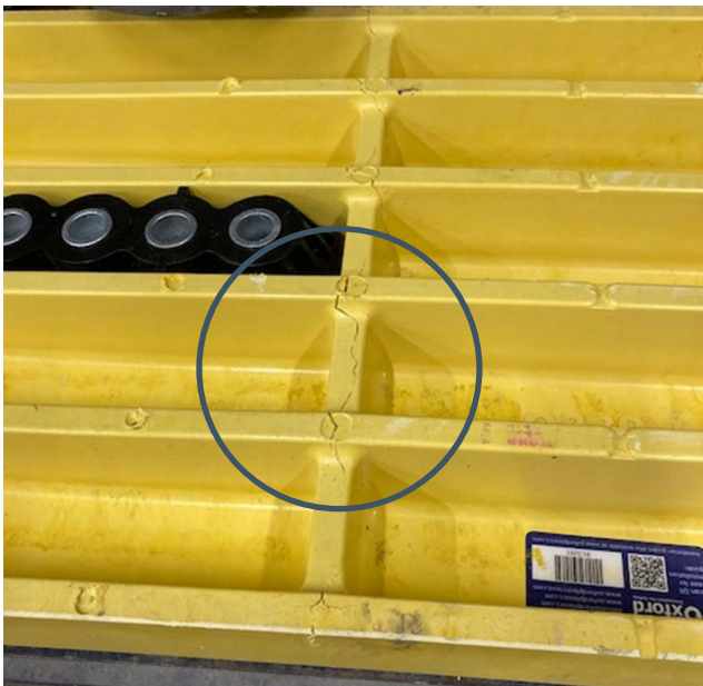
Crack along rib
