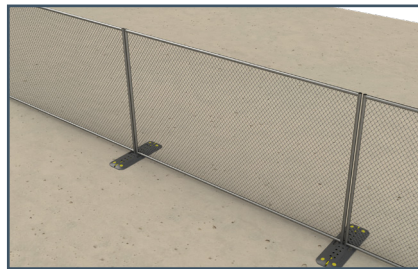
Repeat process until required area is fenced off.
