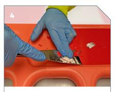
Use the scraper to lift the edges and peel off the damaged reflective.
