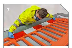
Remove the backing paper from the reflective strip and place it on the barrier, ensuring that it is in the centre of the recess.
