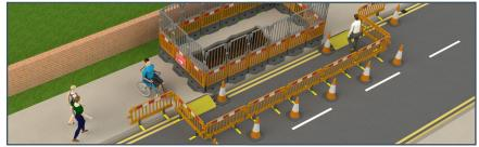
Place a barrier or cone on either side of the pedestrian access route to remove risk of pedestrians not using the access route.
