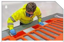
Use the applicator and, applying a firm pressure, work one end to the other in a zig-zag motion pushing down the sticker and removing the air from underneath.
