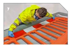
Remove the backing paper from the reflective strip and place it on the barrier, ensuring that it is in the centre of the recess.
