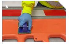
Use a new sponge coated in Standard Primer and, starting at the bottom, ensure that the primer has covered and wetted the whole area. Leave to air dry for 5 minutes.
