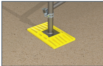
Place scaffolding pole onto the base plate.
